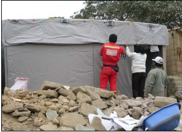
A volunteer firefighter helps community members in southern Peru build temporary shelters with reinforced plastic from USAID/OFDA.
